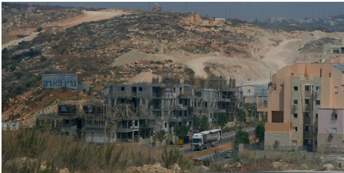
Modi'in Ilit (near Ramallah) – The Canadian company Green Park advertising its properties under construction. August 2010 – Al-Haq©
