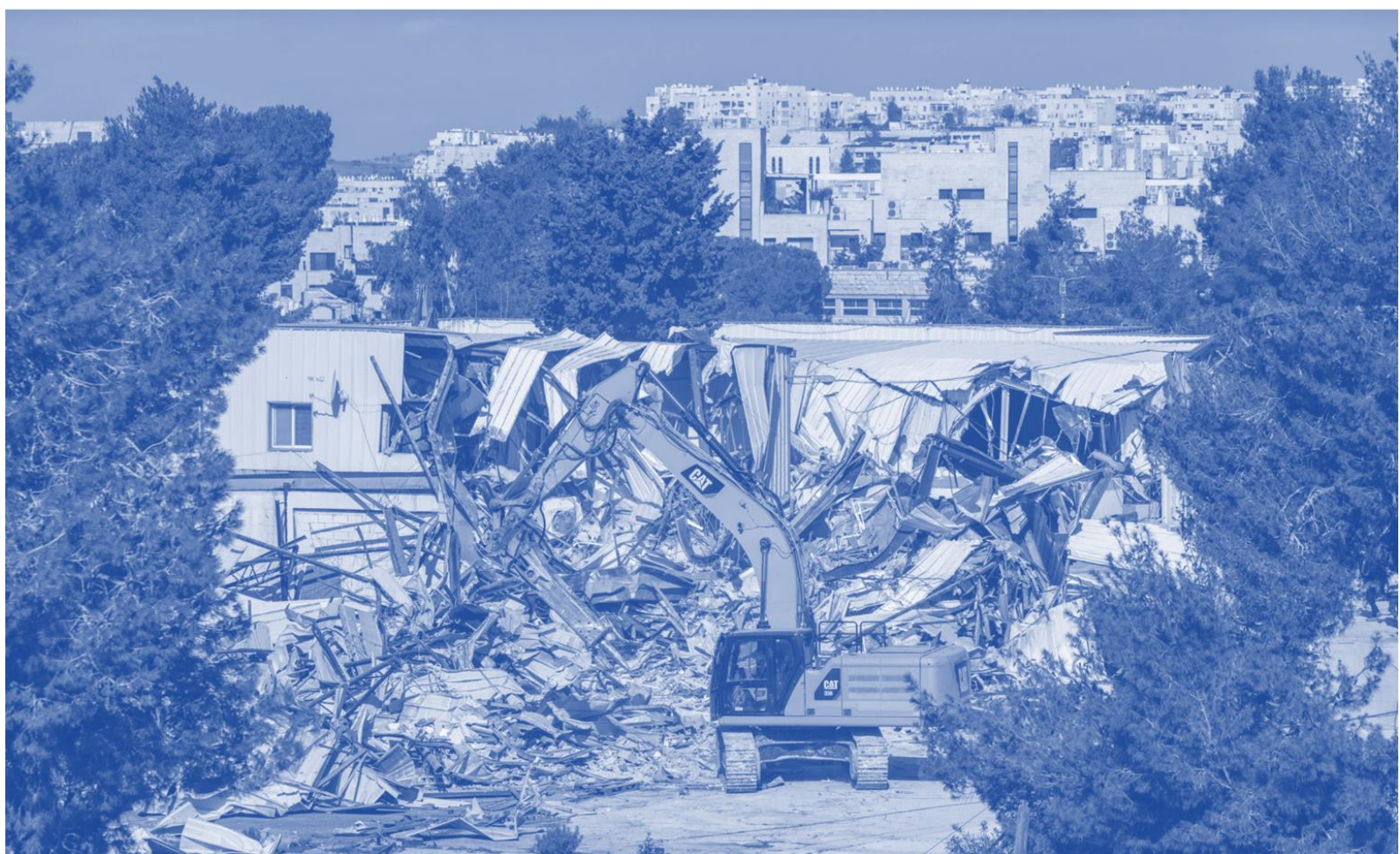
Israeli authorities demolish an UNRWA compound in occupied East Jerusalem (January 20, 2026)
