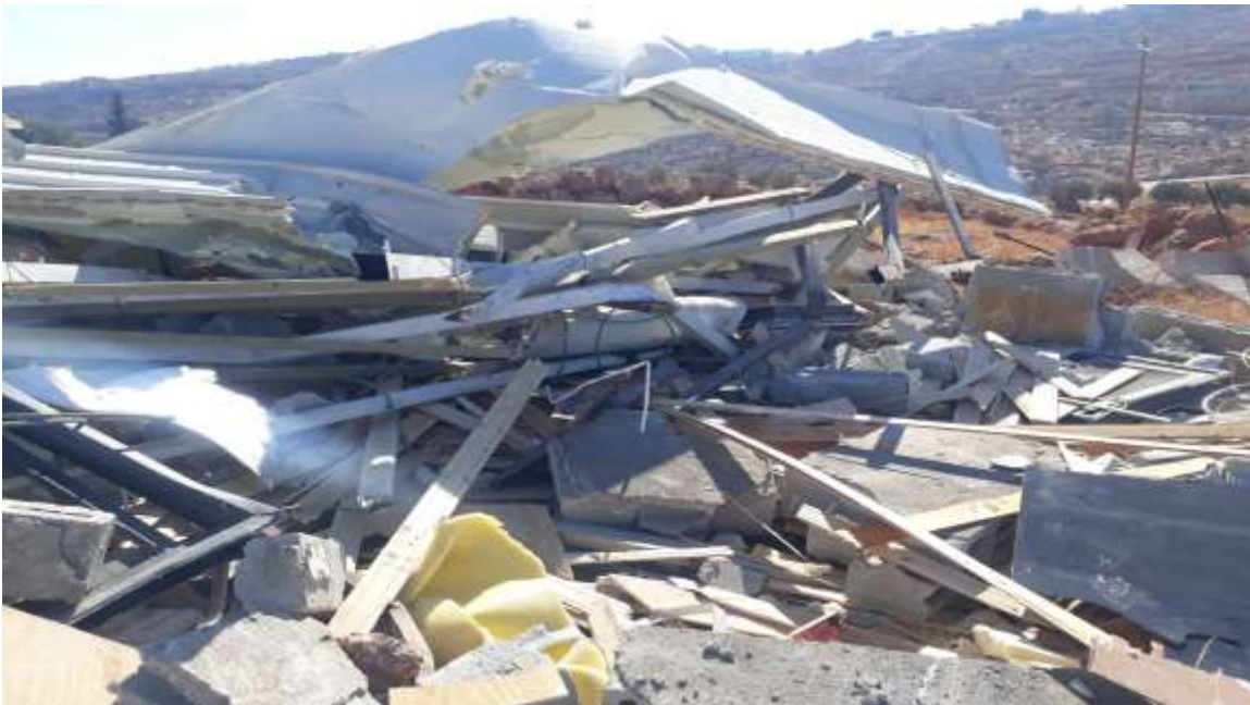
A mosque demolished in Duma, November 2021
