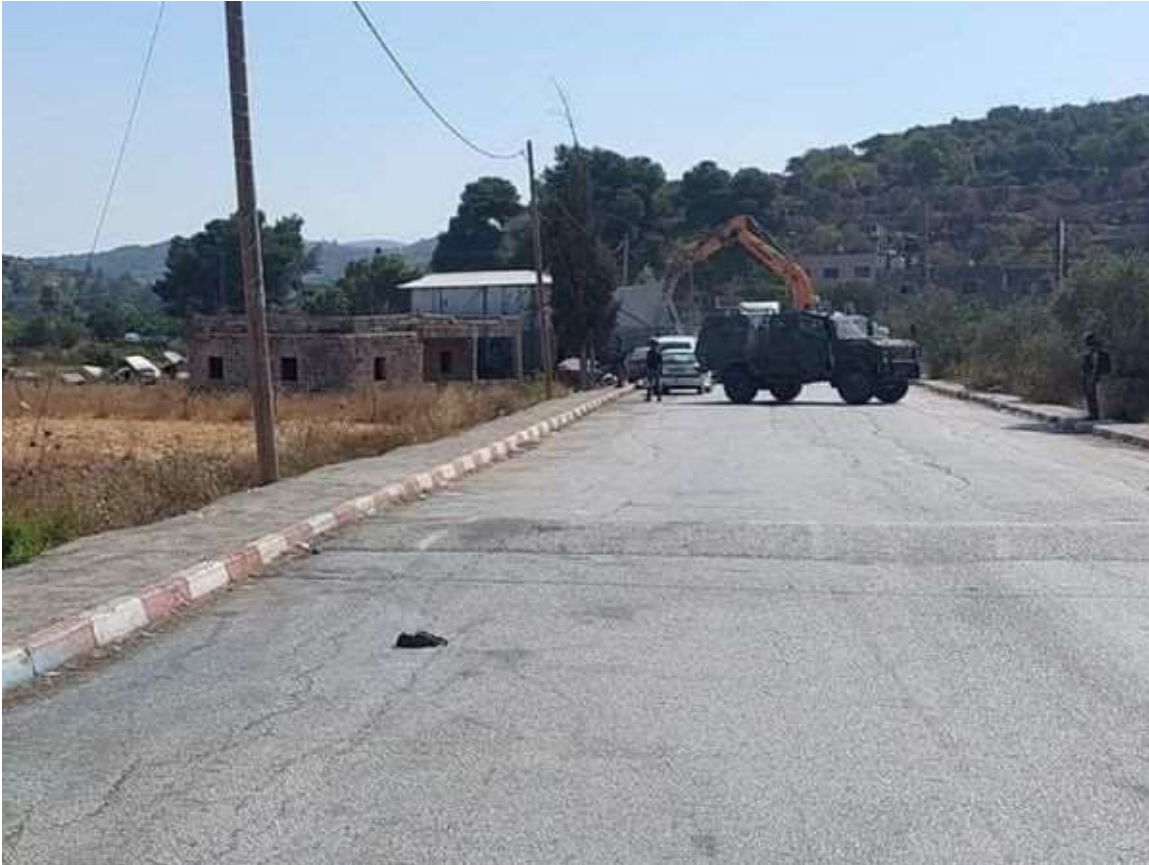
A structure demolished in Al-Lubban al-Sharqiya, August 2021.
