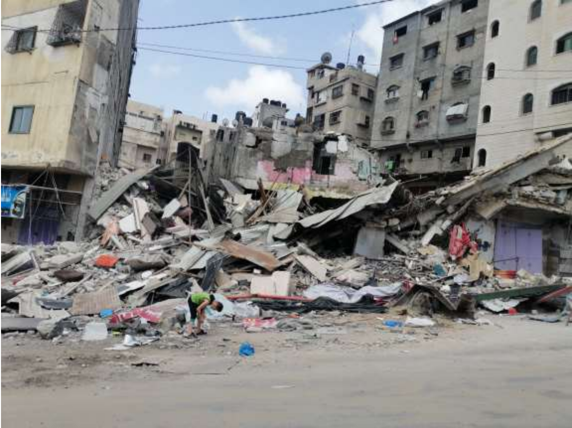
Figure 3: Kuheil building, opposite Al-Shuja'iyah Park, east of Gaza city, destroyed by Israeli warplanes, 20 May 2021
