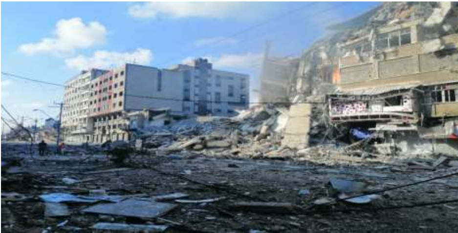
Figure 1: Al-Shurouq Tower destroyed, 13 May 2021, Gaza city.
