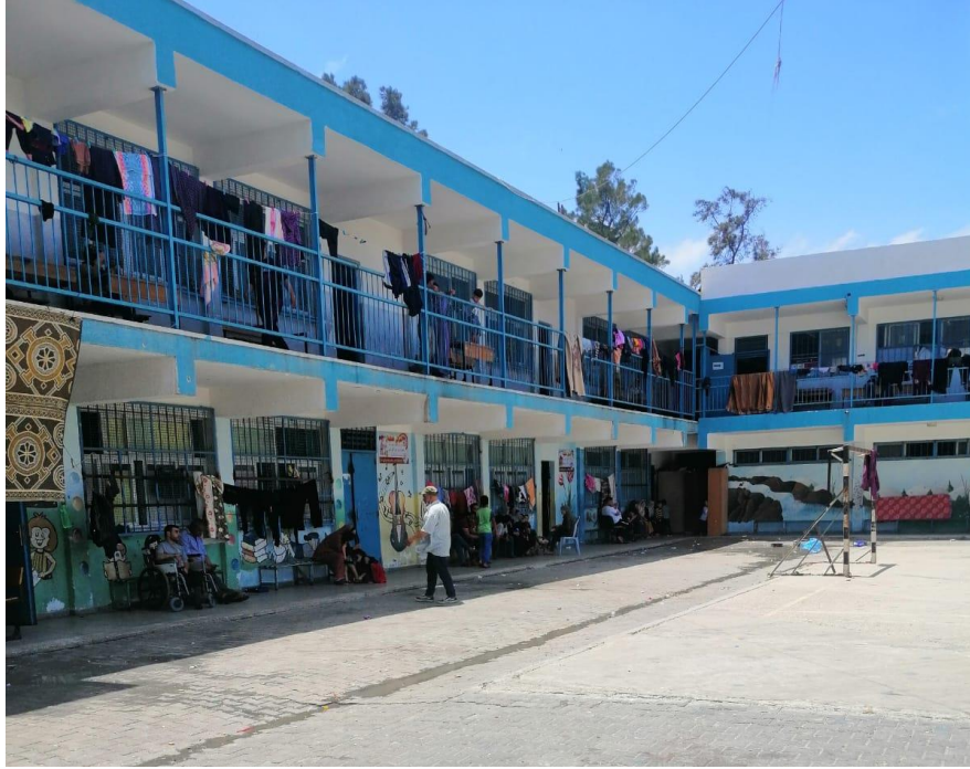
Annex I: Image of UNRWA Boys' Primary School, C and D, designated as a safe haven in Al-Nasr Street, Gaza City. 17 May 2021, on file with Al-Haq.
