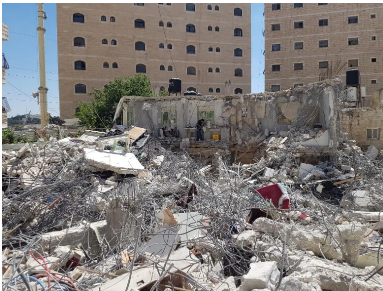
Figure 4: A demolition in Shu'fat refugee camp, June 2020
